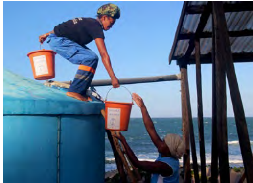
Field agents deep cleaning a 10 000 L water tank. Photo credit: H. Chaplin, Tatirano Social Enterprise.
