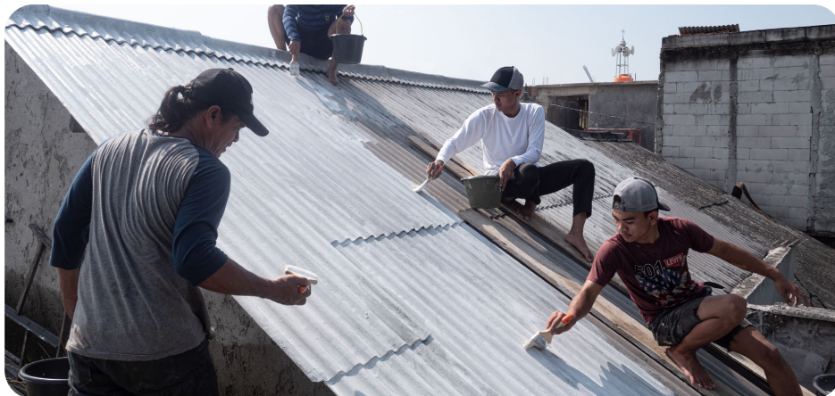
Cool Roofs Indonesia team hard at work (Credit: Clean Cooling Collaborative)
