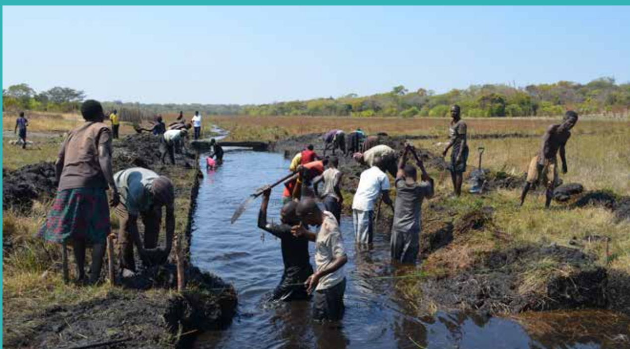
Climate Resilience in Zambia, local people digging out a water channel. © CIF Action
